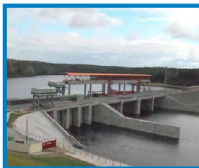
Grodnenskaya HPP / Belarus 5 x Kaplan PIT / 18,870 kW
